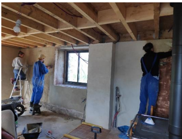
A Les 7 Vents 3SR renovation worksite.
