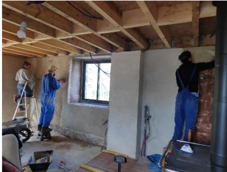
A 3SR worksite.
