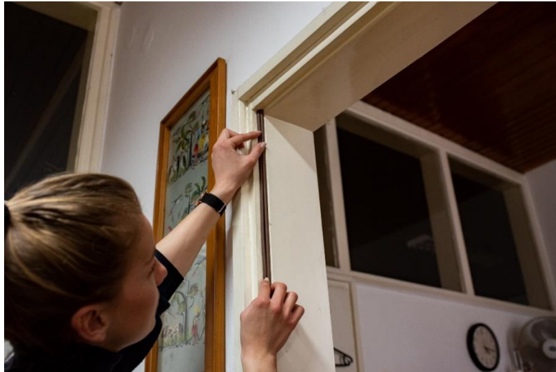
Fitting a draught excluder at a Green Energy Cooperative (ZEZ) home visit.
