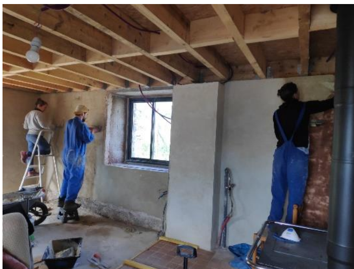
A Les 7 Vents 3SR renovation worksite.
